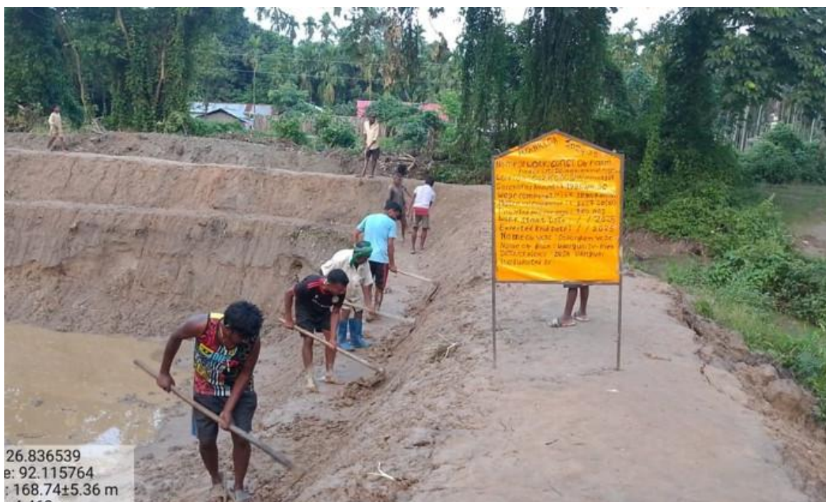
Figure 16: A Farm pond under construction
